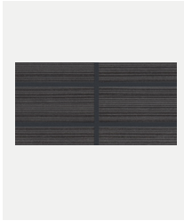
Horizontal Decorative Tile Detail in the Owner's Shower
